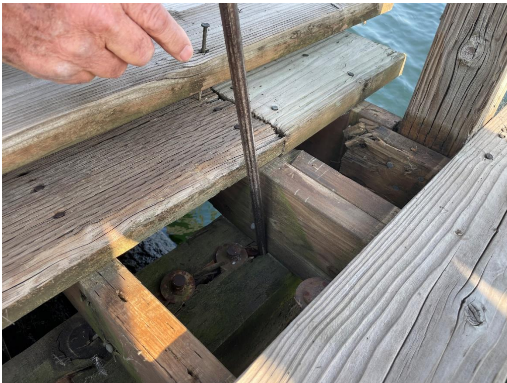
Figure 3 Deteriorated Stringers
