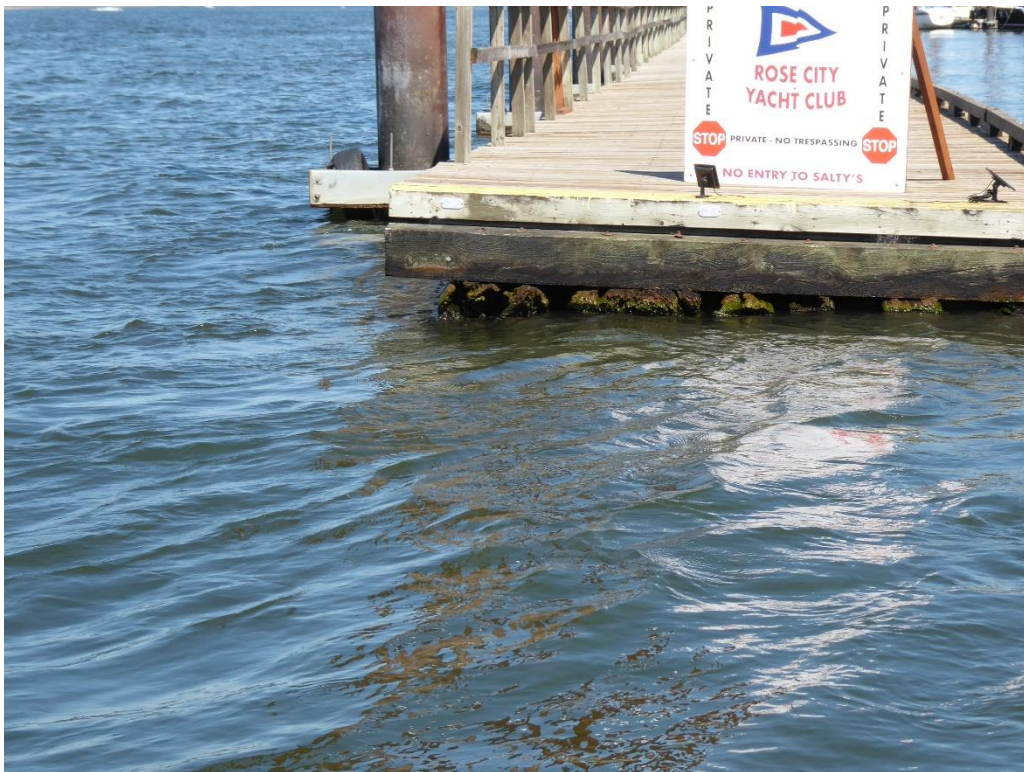
Figure 2 Deteriorated End Condition of Logs
