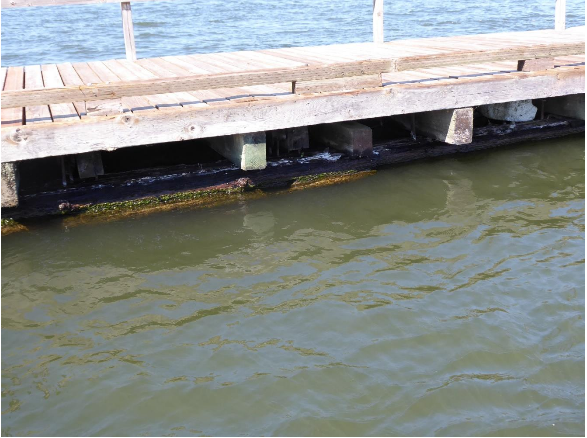
Figure 7 Handrails, Walers and Mooring Beam
