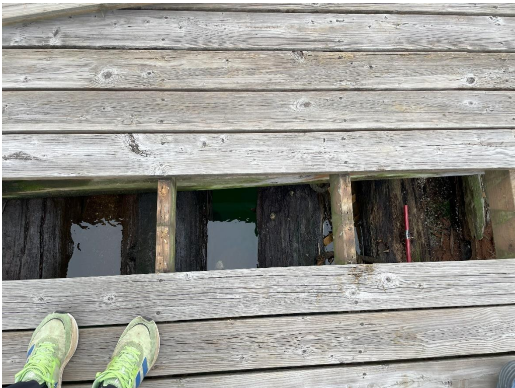
Figure 6 Deteriorated Logs with Coring Tool
