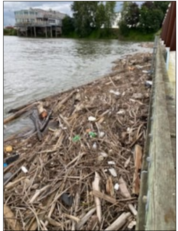
Debris accumulating during high river levels against the upriver side of Walk 1
