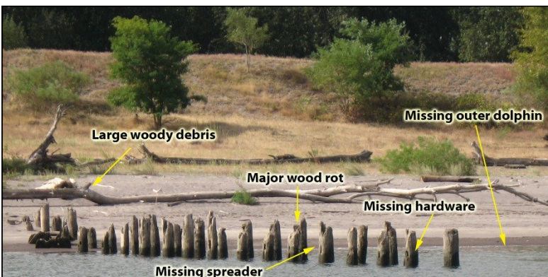
Wingdam hazard you don't see when river levels are higher
