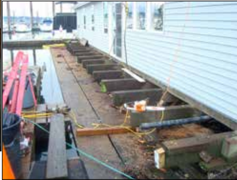
Work has started.
