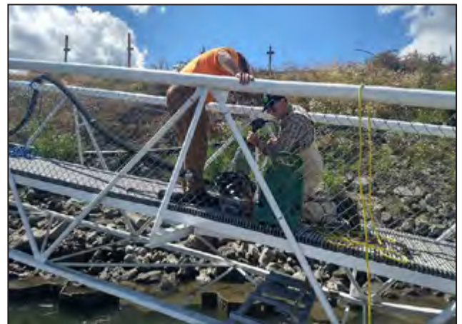
Tom Stringfield working with Martin Foster to fix water line feeding water to the marina.
