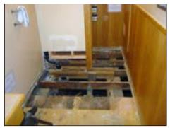
The rotten flooring has been removed and waiting for new pressure tread plywood to be installed.
