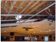
The rusted "T" bars and water spotted ceiling panels have been removed.
