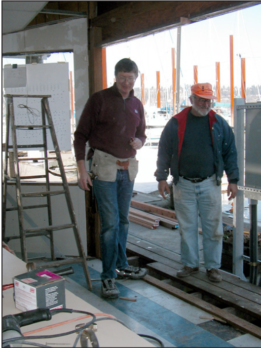
2004 Clubhouse remodel - it took many hands, many hours, and great team work.
