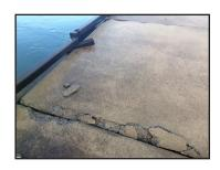
Logs or other waves have slammed into the transient tie-up at Sandy Beach and broke a 40 foot section of dock. Currently the rest of the transient tie-up is still accessible.
