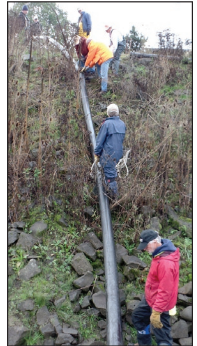
RCYC crew assembling the dredge discharge pipe.
