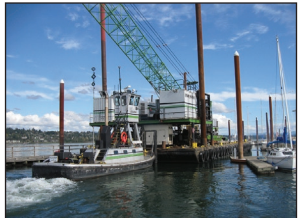
Walk 2 and 3 piling project
