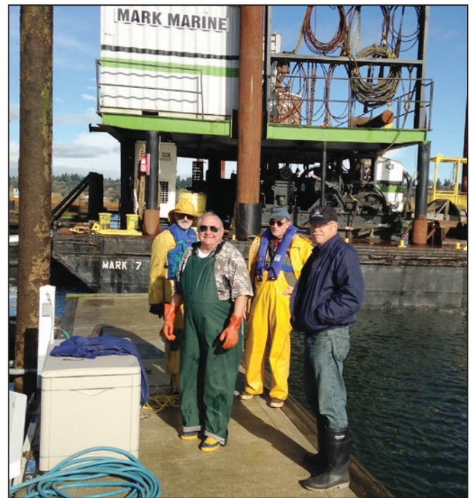
November RCYC calendar men? Na, part of your piledriving and dredge crew: Bob Fellman, Jim Hackley, Tom Stringfield, and Brad Jensen.
