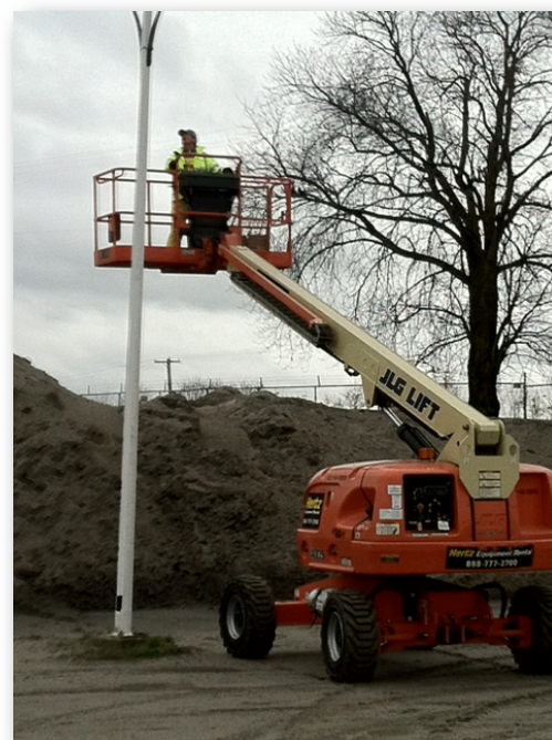
Dave Kibby doing electrical repairs
