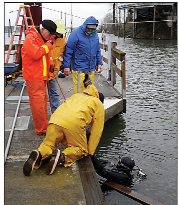
Retrieval of the Dredge Outflow pipe on 12-29-2010. Terry (diver) worked in the COLD river water to locate and put a sling on the broken off piece of dredge pond outflow pipe. RCYC could then pull the piece of pipe to a manageable position and tie it off. Pipe piece will be reattached in warmer weather.
