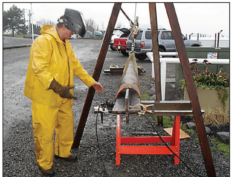
Fabrication of the dredge's new left spud pipe: Brad Jensen, Tom Stringfield, and Ron Billion.
