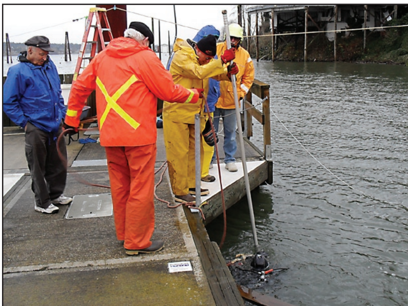
Retrieval of the Dredge Outflow pipe on 12-29-2010. Terry (diver) worked in the COLD river water to locate and put a sling on the broken off piece of dredge pond outflow pipe. RCYC could then pull the piece of pipe to a manageable position and tie it off. Pipe piece will be reattached in warmer weather.
