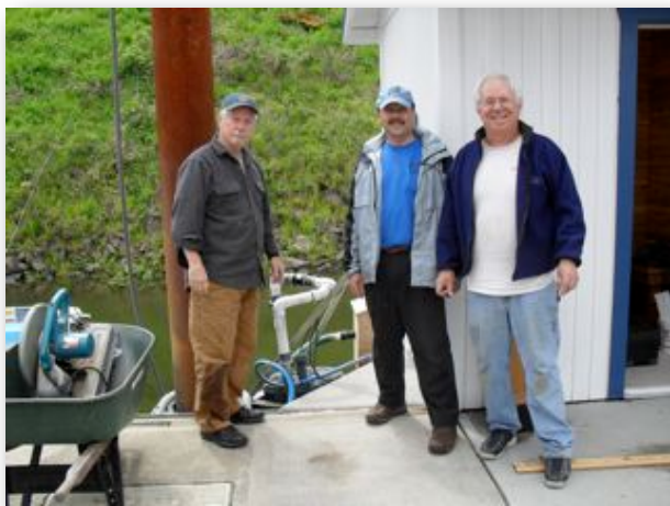
Special work crew finishing shower connections
