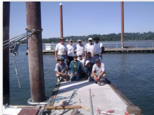
Work crew installed final walk 5 section
