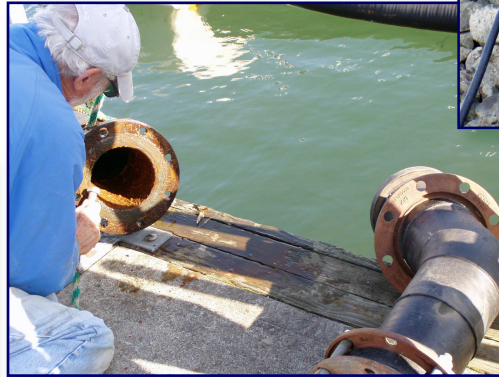
Dredge Pipe Inspection, Mike Pick
