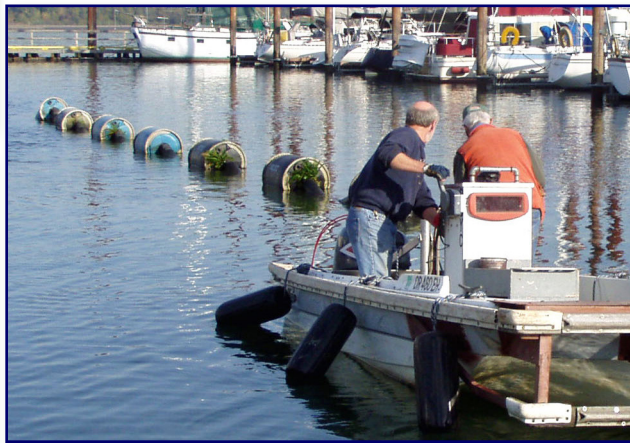
Floating the Dredge Pipe, Larry Wintermeyer and Terry Foren
