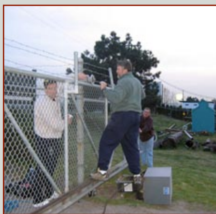
Ron Billion and Lynn Easton working to get the gate operational again.
