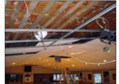
The rusted "T" bars and water spotted ceiling panels have been removed.
