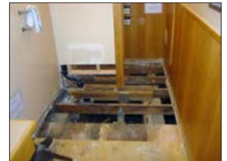
The rotten flooring has been removed and waiting for new pressure tread plywood to be installed.
